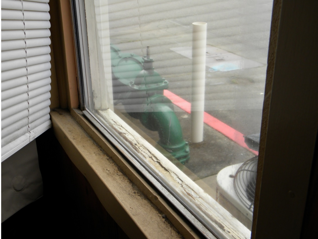
#7 Dry rot window sills station #31
