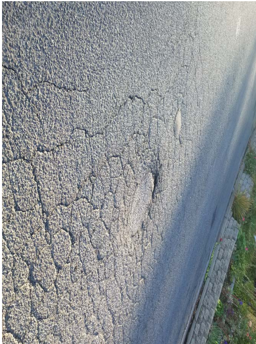
Figure 3: Example of street deterioration with pothole and alligator cracking
